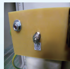
Specific Grounding Screw
