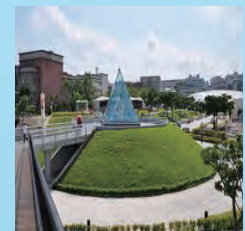
Park Electric Equipment
